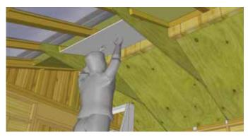
**11.** Locate and position center ceiling plywood panels below Rafter and Short Roof Cleat. Attach panel to Rafter and Gable Cleat with **8 - 1 1/4" screws**. Complete three panels.
