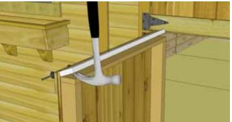
**27.** To accomodate Interior Door Plywood, the existing top plate on bottom door must be removed first. Using a hammer, carefully pry off the top plate and remove any hardware.
