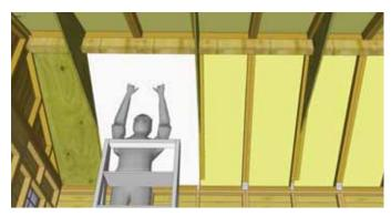
7. Locate and position center ceiling plywood (44 3/4" wide) panels and position against Rafters and Roof Cleats. When positioned correctly, attach to Rafter and Roof Cleat with 12 - 1 1/4" screws. Complete three sections.
