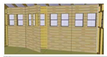
19. Locate Double Window Wall Center Panels (45 1/4" wide). Panel wall siding will be flush with plywood backing. Position between previously installed panels on wall studs and secure with 6 - 1 1/4" screws per panel. Complete both panels.
